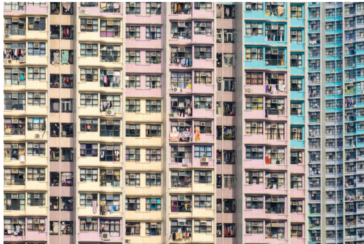
Public Housing Block New Territories Hong Kong China Photograph
